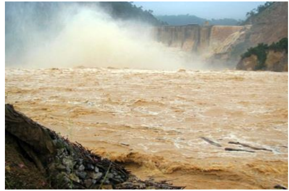
Figure 1. Water spilling over top of Ho Ho dam due to uncontrollable flood.
